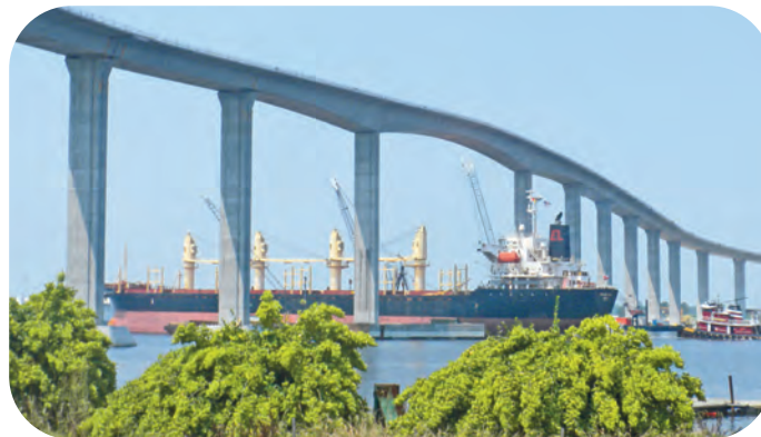
South Norfolk Jordan Bridge, Virginia
