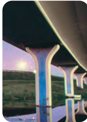
Rounded Pier Selmon Expressway, Florida
