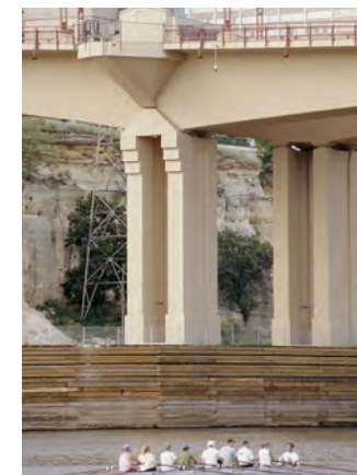
Angular Pier Wabasha Freedom Bridge, Minnesota
