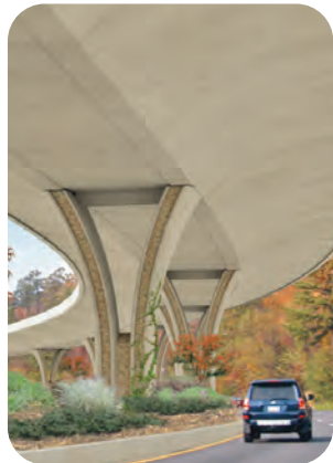
Curved/Open pier US 280 Elevated Roadway, Alabama
