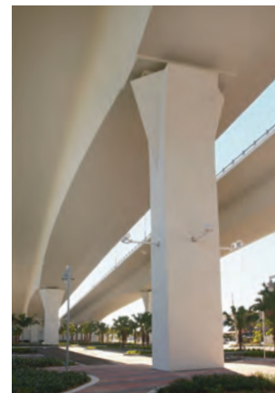
Angular Slender Pier 17th Street Bridge, Florida
