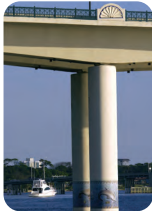
Elliptical Pier with Glass Mosaic Tiles Broadway Bridge, Florida
