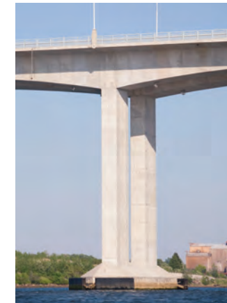
Angular Pier Victory Bridge, New Jersey
