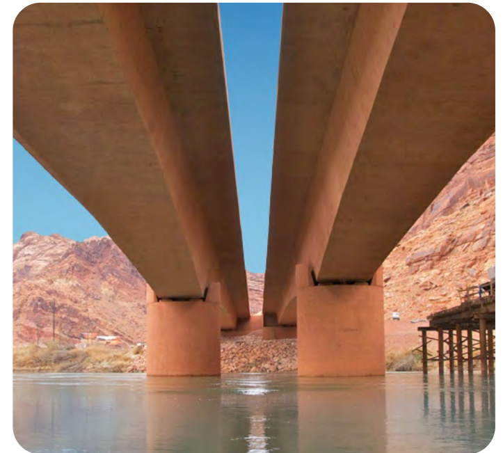
US 191 Colorado River Bridge, UT
