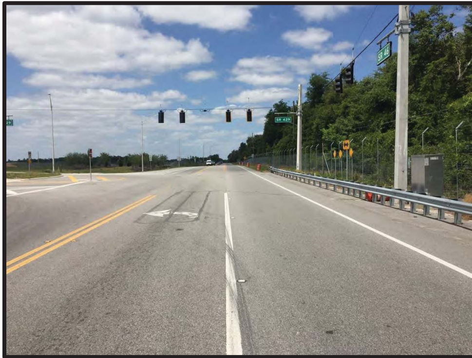
Looking West Towards Intersection
