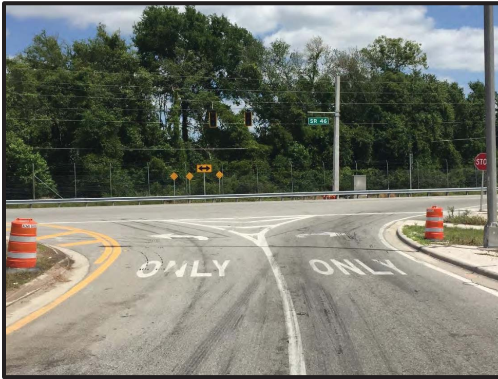
Looking North Towards Intersection
