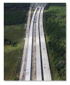
The wildlife bridges (*photos, left and below*) have replaced the former wildlife tunnels in the Rock Springs Run State Reserve. The previous tunnels had about 80 feet of clearance for animals to pass under S.R. 46. The new wildlife bridges will total nearly 7,700 feet in length, providing nearly 100 times the safe passageway for animals as the previous tunnels. All told, Section 6 involves driving approximately 1,900 concrete bridge foundation piles.
