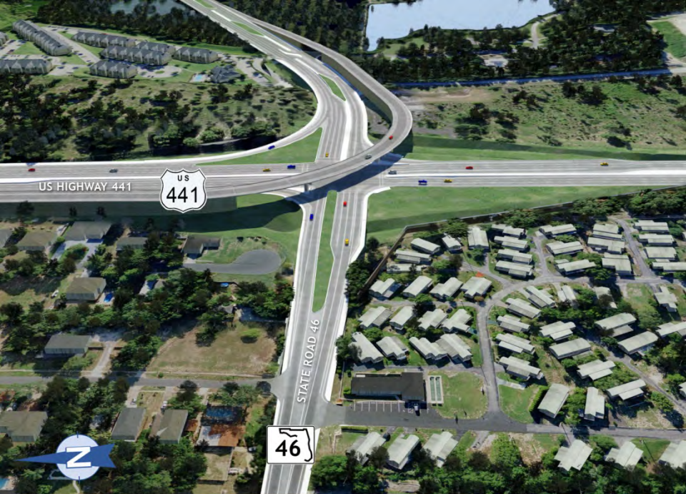
AT GRADE INTERSECTION WITH FLY-OVER BRIDGE – EASTBOUND VIEW
