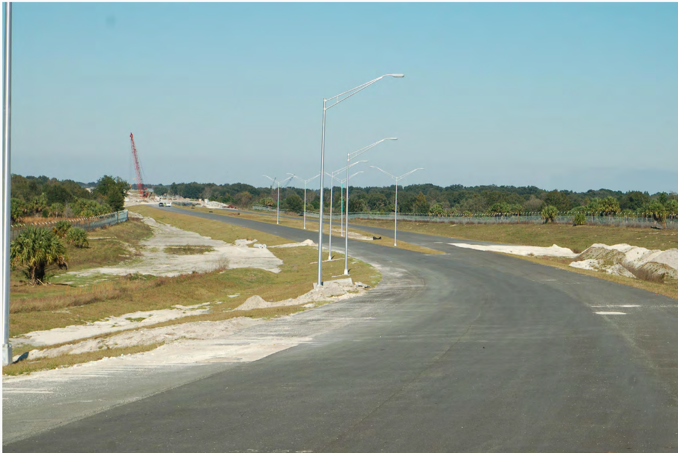
Pavement, street lights and wildlife fencing on Section 4A near CR 435 (Mt Plymouth Road)
