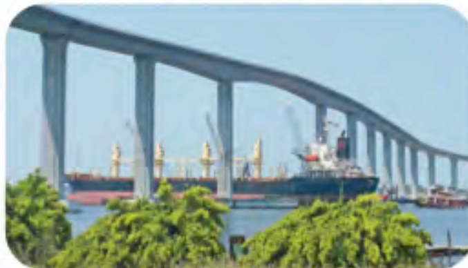
South Norfolk Jordan Bridge, Virginia
