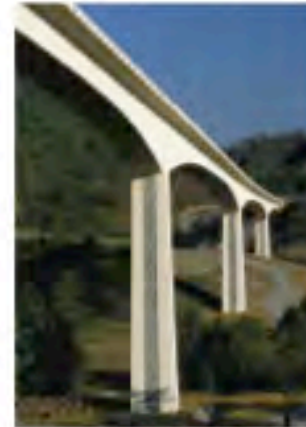
Tapered Pier with Local Stone Smart Road Bridge, Virginia
