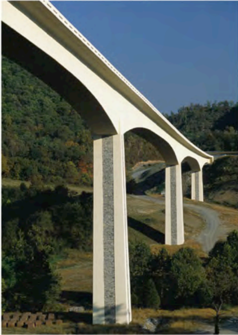
Smart Road Bridge, Virginia
