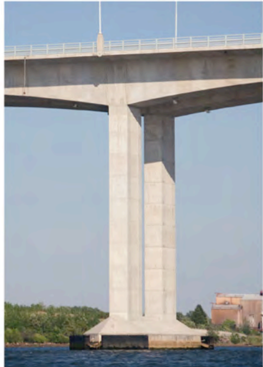
Victory Bridge, New Jersey
