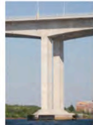
Angular Pier Victory Bridge, New Jersey
