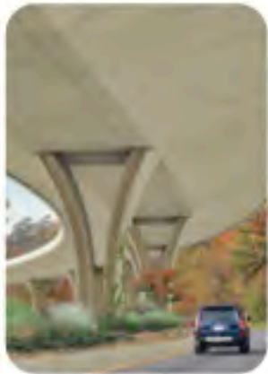
Curved/Open pier US 280 Elevated Roadway, Alabama
