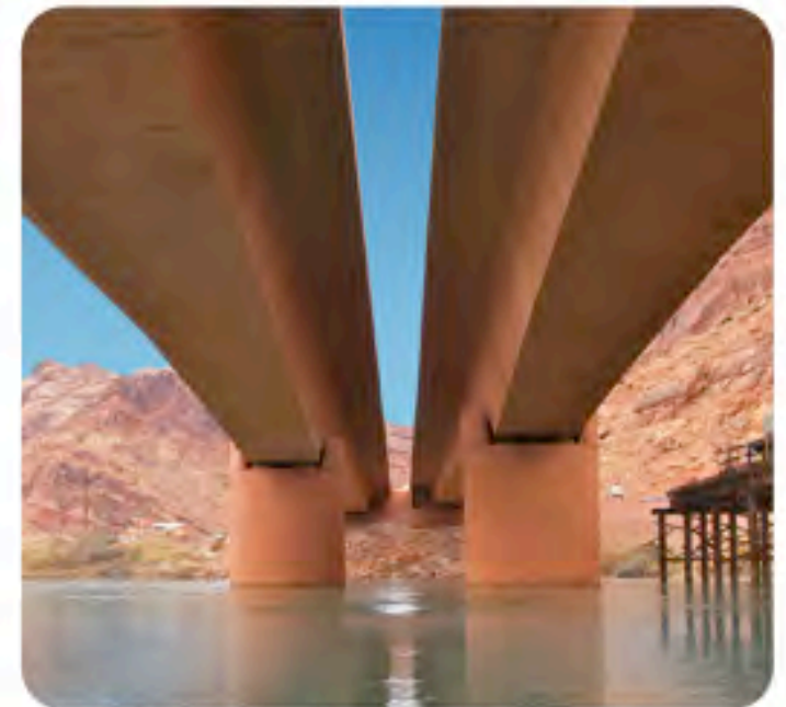
US 191 Colorado River Bridge, UT
