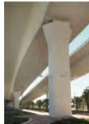
Angular Slender Pier 17th Street Bridge, Florida
