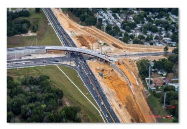
Work continued to build the new flyover bridge columns and retaining walls. The structures feature the characteristic parkway stone relief and will be painted in warm browns and tans to give a more natural, rustic appearance. Flyover bridge beams will be painted deep green to help blend into the surroundings.
