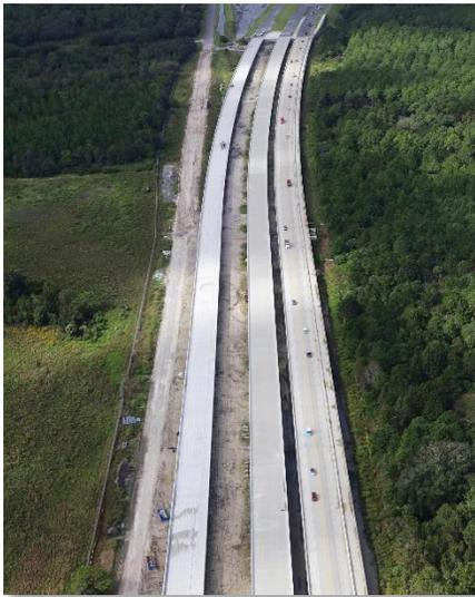
The wildlife bridges (*photos, left and below*) have replaced the former wildlife tunnels in the Rock Springs Run State Reserve. The previous tunnels had about 80 feet of clearance for animals to pass under S.R. 46. The new wildlife bridges will total nearly 7,700 feet in length, providing nearly 100 times the safe passageway for animals as the previous tunnels. All told, Section 6 involves driving approximately 1,900 concrete bridge foundation piles.
