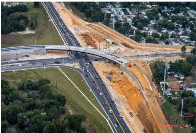
Work continued to build the new flyover bridge columns and retaining walls. The structures feature the characteristic parkway stone relief and will be painted in warm browns and tans to give a more natural, rustic appearance. Flyover bridge beams will be painted deep green to help blend into the surroundings.
